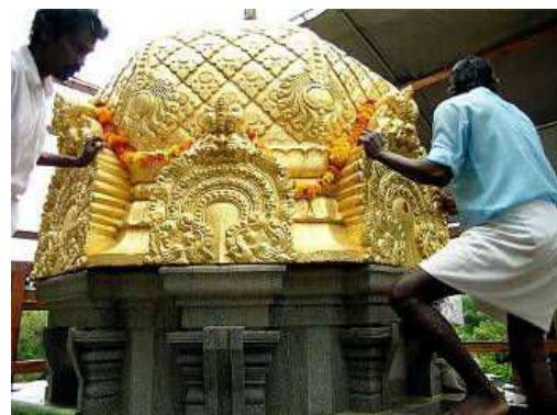
Figure 48 –The process of placing the cap stone or sikhara (Source: www.himalayanacademy.com )
