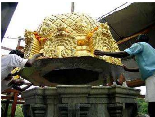
Figure 48 –The process of placing the cap stone or sikhara (Source: www.himalayanacademy.com )
